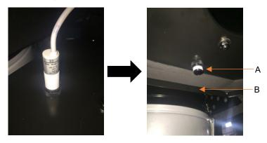
Step 34: Attach the LED light to the drum lid using (6x) M4\*10mm bolts, (6x) 3/16" washers and (6x) M4 nuts.
